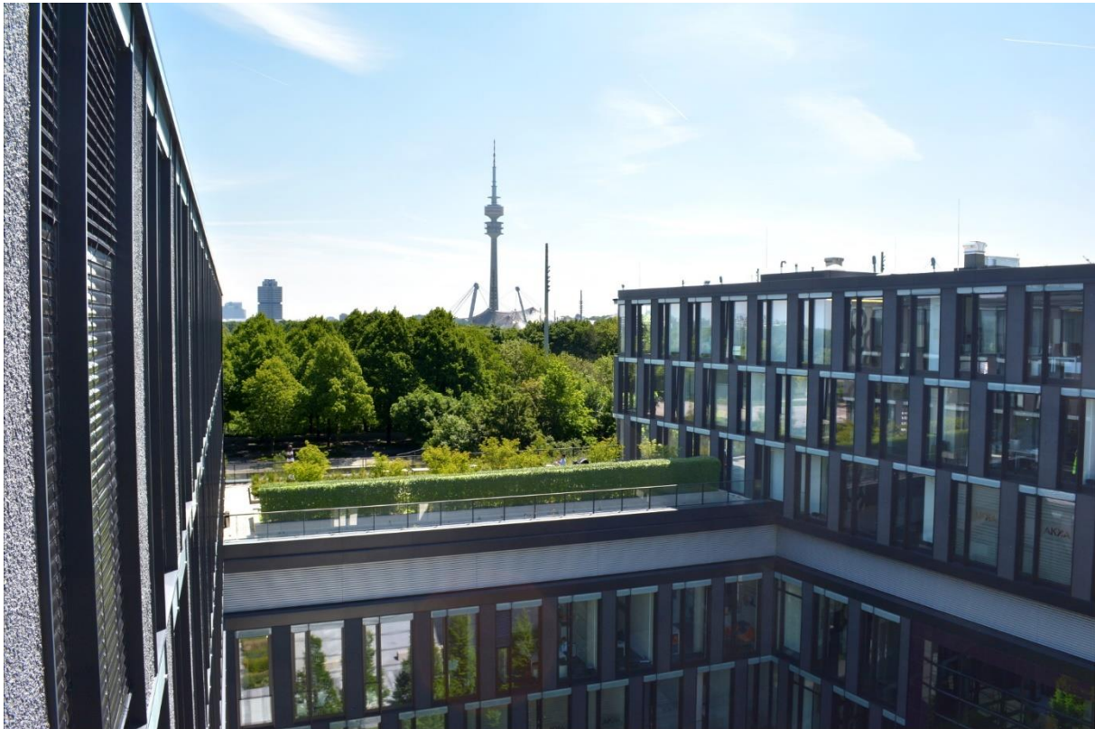
Picture 1: New Logivations´ headquarters in 88 North at the Olympiapark
